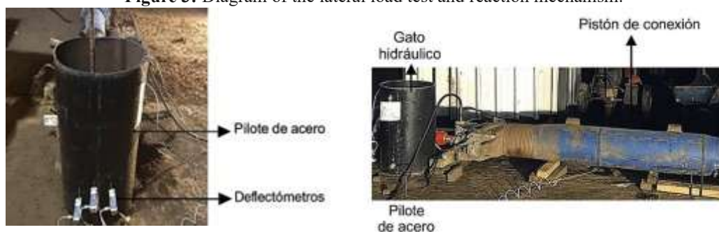
Figure 4: a) Digital strain gauges at the pile head and b) connection mechanism.
